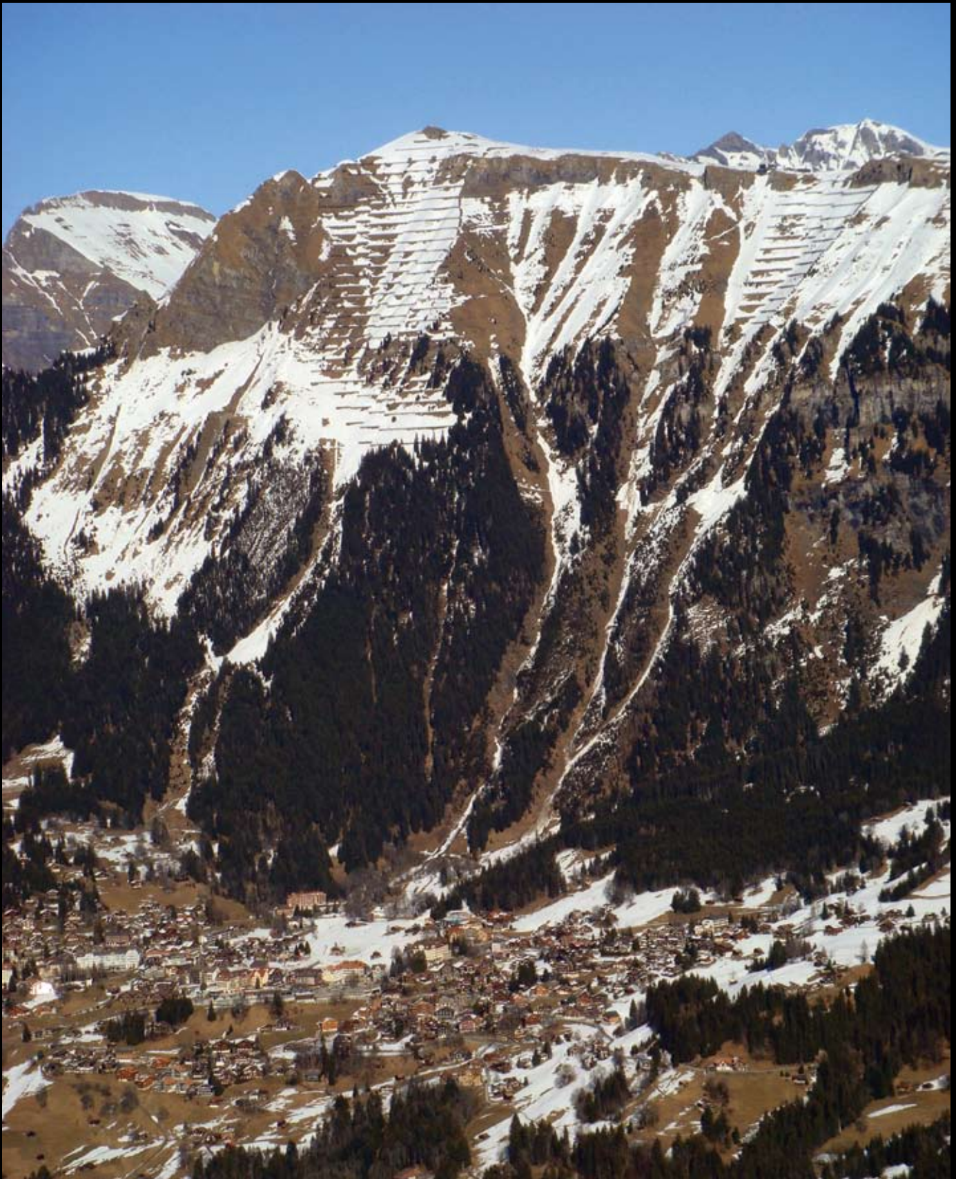
Spring in Wengen, Switzerland. Between the avalanche tracks, which reach all the way to the village, spruce forests serve as protection. Above the forest line, protective barriers made out of steel and wood prevent the scribing of avalanches.
